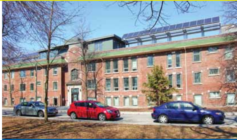
Toronto Community Housing - Regeneration of Rental Housing Contractor: Lisgar Construction Company Architect: Van Elslander Carter Architect Incorporated
