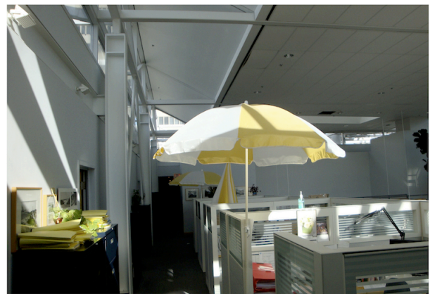
Figure 2: Existing 3 rd Floor Glare Control Devices
