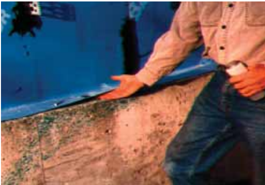
Figure 10: Membrane is not sealed to the substrate.
