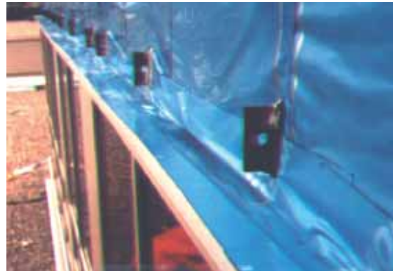
Figure 11: Bad workmanship at window frame.
