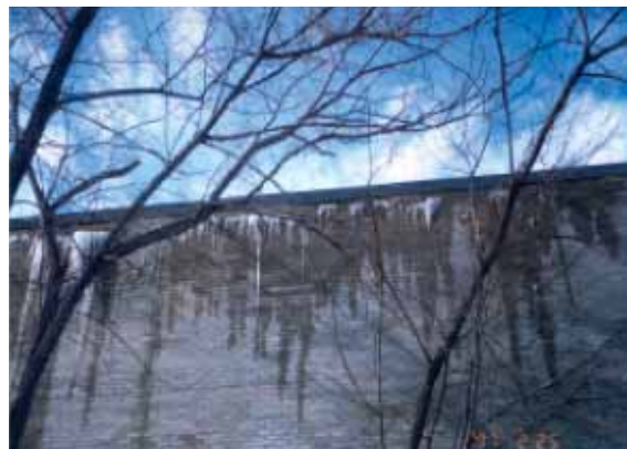
Figure 2: Ice forming on exterior of building.
