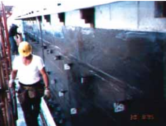
Figure 7: Masonry being installed immediately after a section of air barrier.
