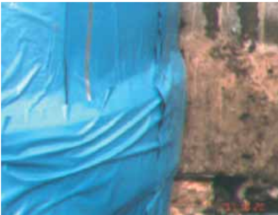
Figure 8: Flutes in an air barrier membrane.
