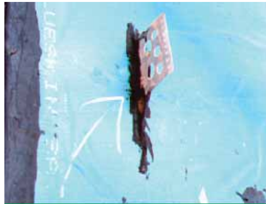
Figure 9: Membrane is not sealed at the penetration.
