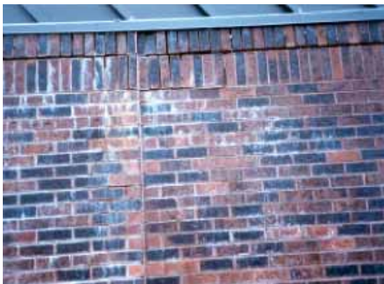
Figure 1: Efflorescence and spalling of bricks and mortar.
