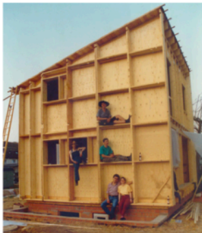
Das Minimalhaus | Stuttgart, Germany, 1996
