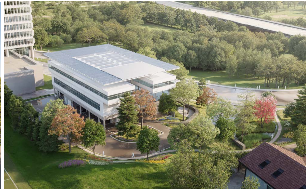
Aerial view from the south-west
