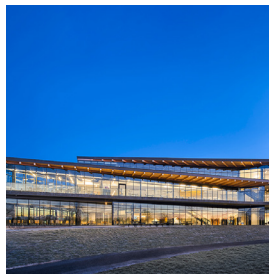
Trent University Student Centre (Peterborough, Ont.) Teeple Architects Inc.
